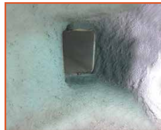
Chamber Coat Application Seals Gaps, Cracks, Holes, and Streamlines Smoke Chamber Walls
